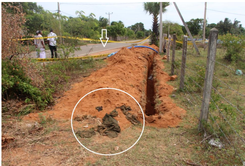
Figure 2: The site of initial excavation adjacent to B-297 road (arrow), which led to the discovery of human remains and clothing (circled).
